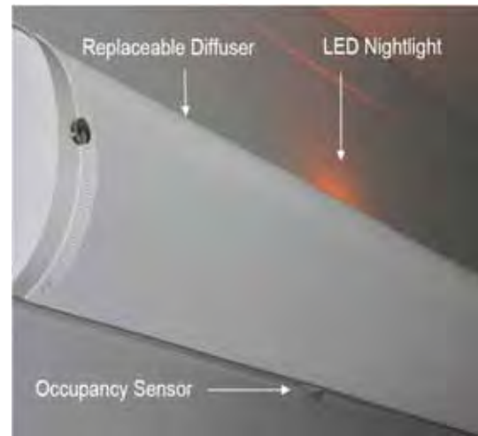
LED Night Light in Hotel Bathrooms
