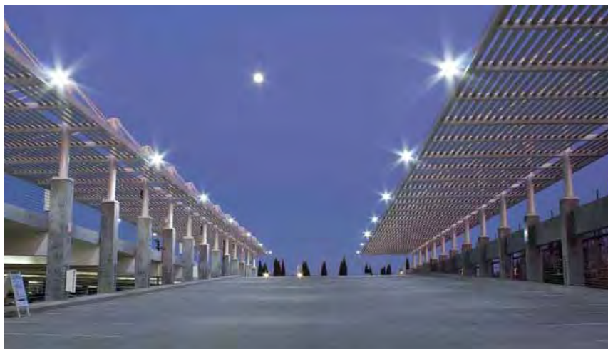
Bi-level Smart Parking Garage Lighting at UC Davis
