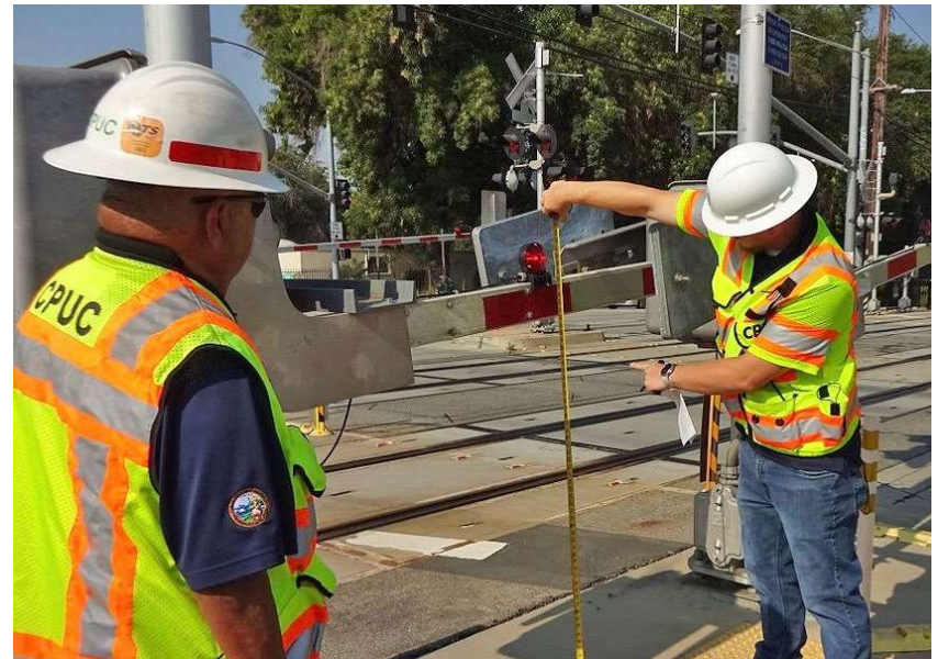
CPUC staff conduct an inspection of the California Boulevard rail crossing on L.A. Metro's A Line in Monrovia, California, on July 9, 2024, verifying that warning devices are in compliance with applicable rules and regulations.
