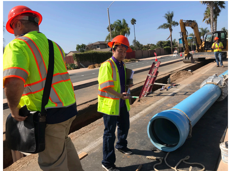
Staff monitors main replacement to ensure reliable water delivery.
