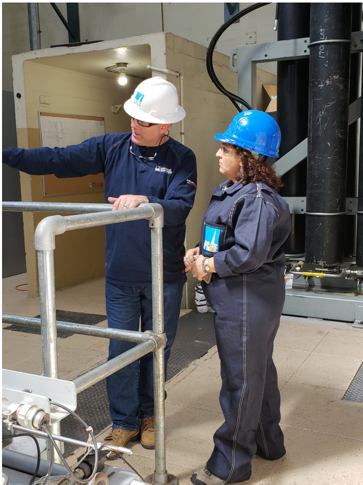
Staff inspection at PG&E.
