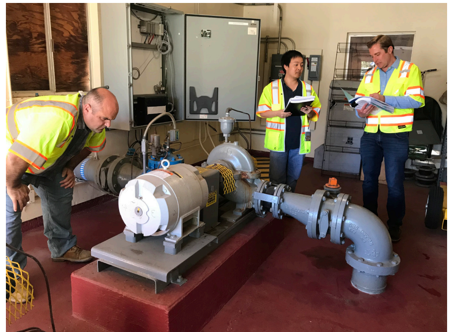
Staff inspects Booster Station so you have fresh clean water when you need it.
