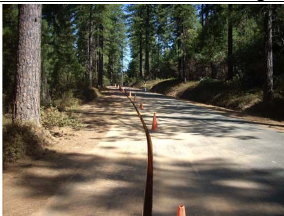
Left photo: trenching for copper cable and conduit for future fiber deployment. Right photo: chip seal on road after trench is filled in.
