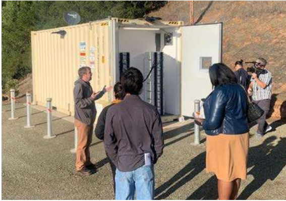
Ribbon cutting for PG&E's Pepperwood Preserve Remote Grid Project
