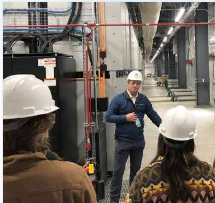
Tour of Moss Landing Power Plant.
